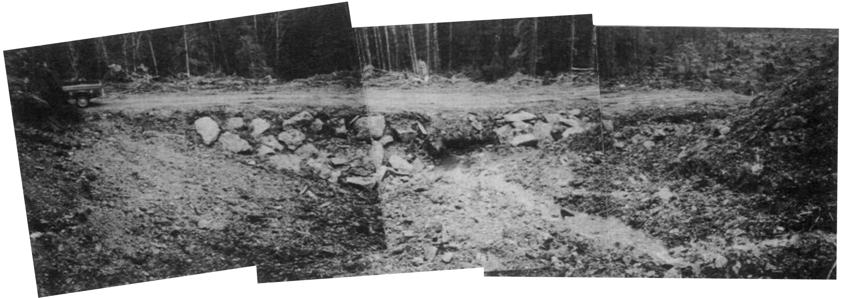
Looking downstream towards terminal berm. Note armoring.
