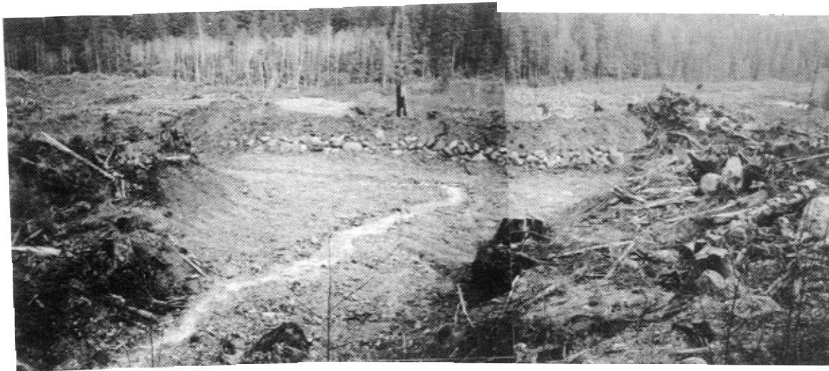
Looking downstream from apex of debris basin towards terminal berm. For scale, berm is approximately 5 m high. Note armouring of upslope side of berm.
